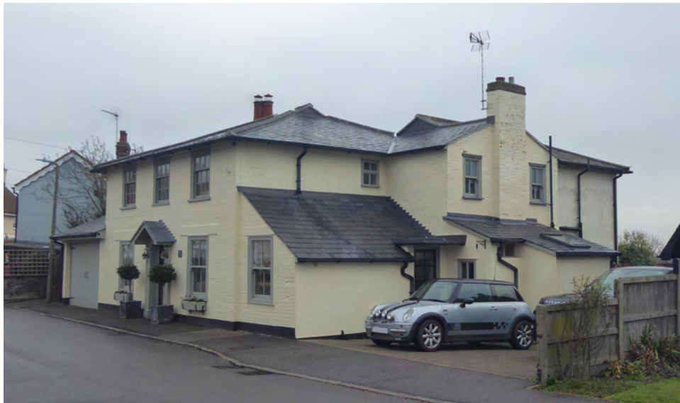
Figure 28 The Saltings, Manor Road
