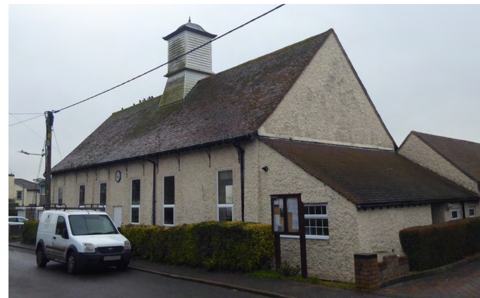
Figure 27 The Village Hall Manor Road
