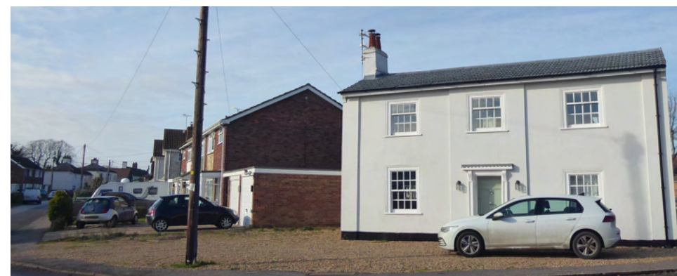
Figure 51 Parking in areas in front of dwellings
