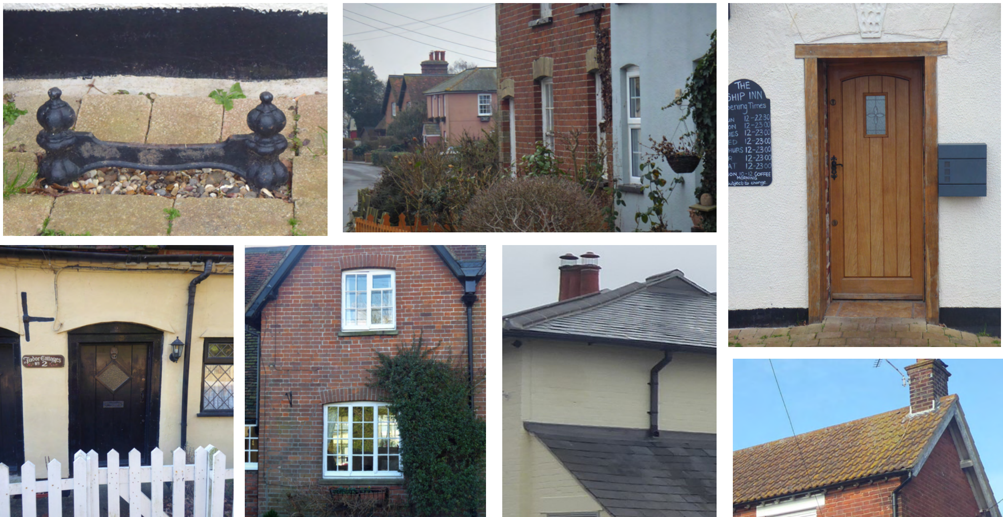
Figure 22 Render, brick, an iron boot scraper, timber doors and windows, slate tiles and clay tiles within the Conservation Area
