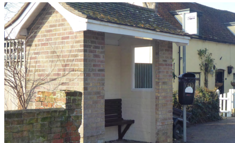
Figure 52 The bus shelter on Rectory Road
